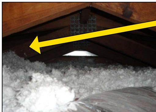
Insulation blown to bottom of trusses w/o baffles
