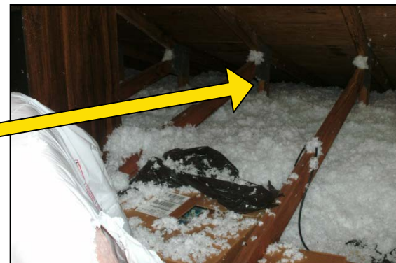
Ducts not strapped to trusses, buried in insulation
