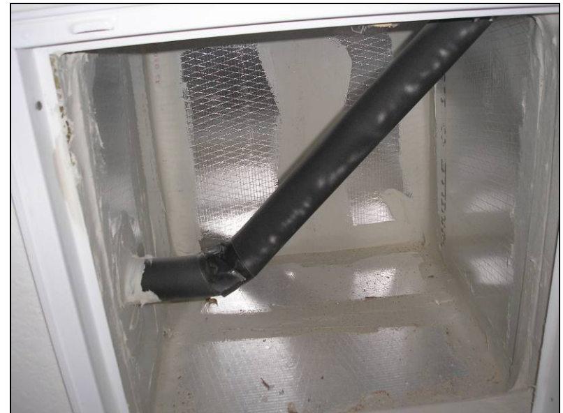
Central return plenum constructed with duct board & sealed with mastic at edges, seams, & joints.
